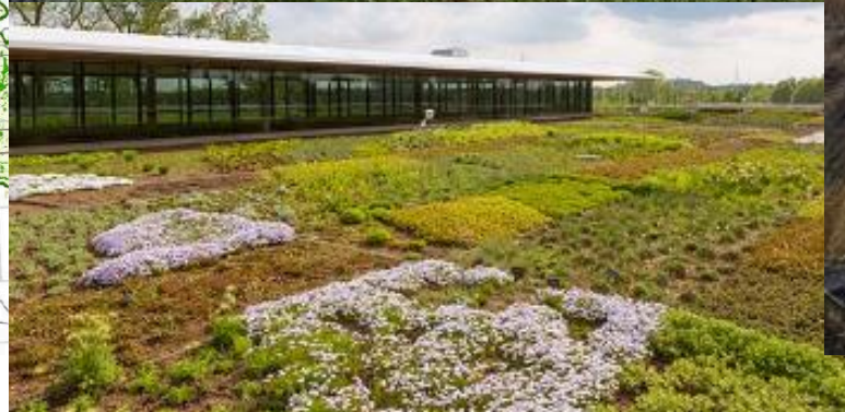
Indian Boundary Prairies, CBG Green Roof Garden
