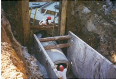
*Photo of open cut sewer installation*
