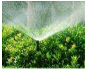
Locations where cross connections may occur in the home: hoses left in laundry sinks & buckets and in underground sprinkling systems
