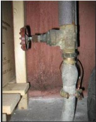
Lead service lines can be connected to the residential plumbing using solder and have a characteristic solder "bulb" at the end, a compression fitting, or other connector made of galvanized iron or brass/bronze.
